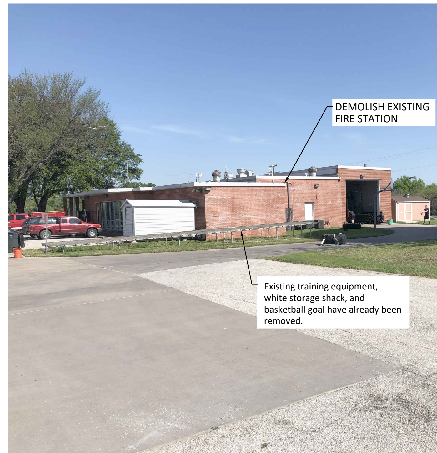
2 FIRE STATION #3 (BACK VIEW)
