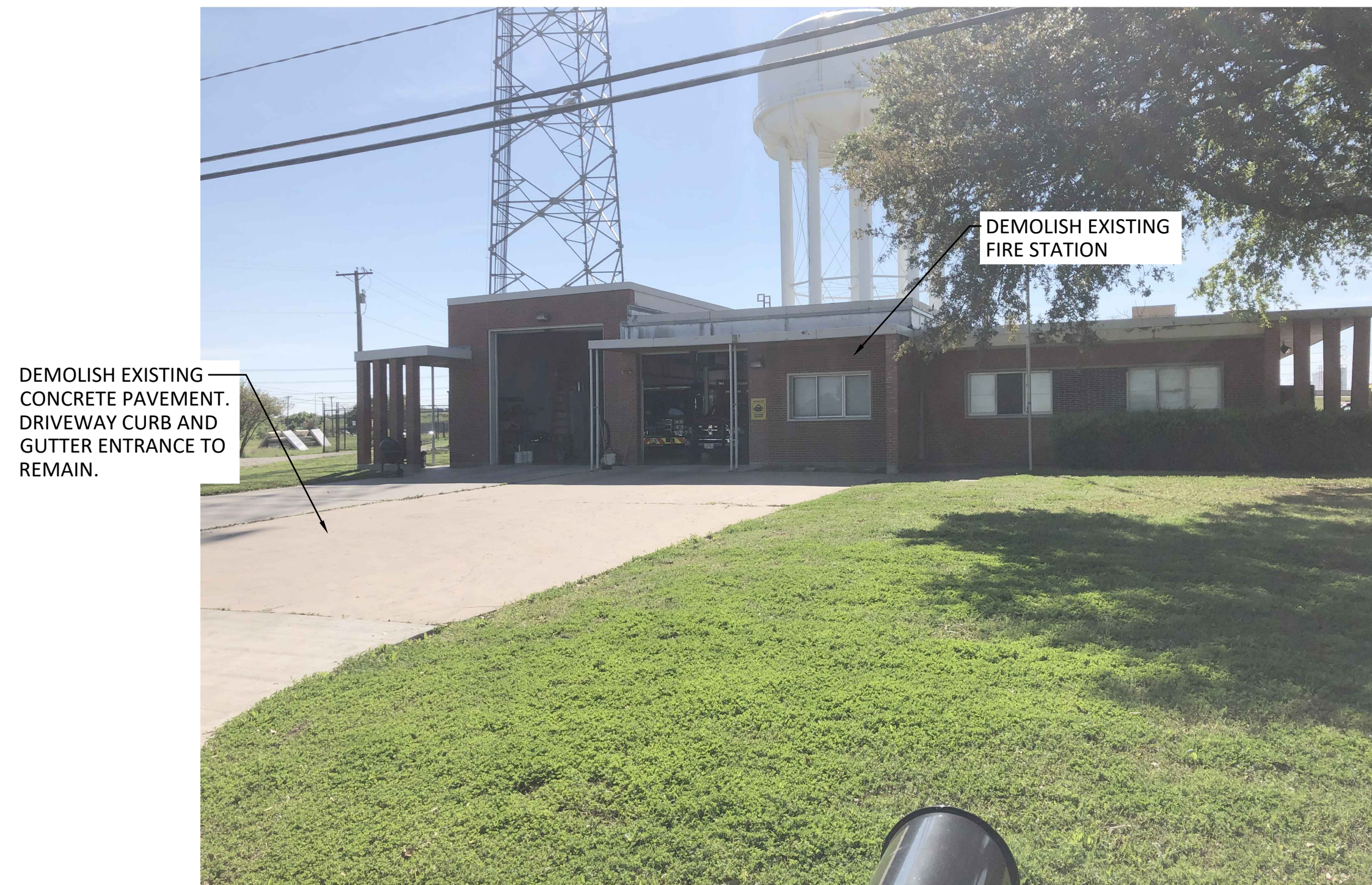
1 FIRE STATION #3 (FRONT VIEW)
